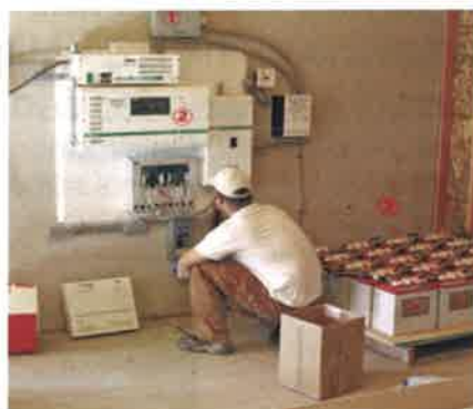
Control System a Hybrid Solar-Diesel System
